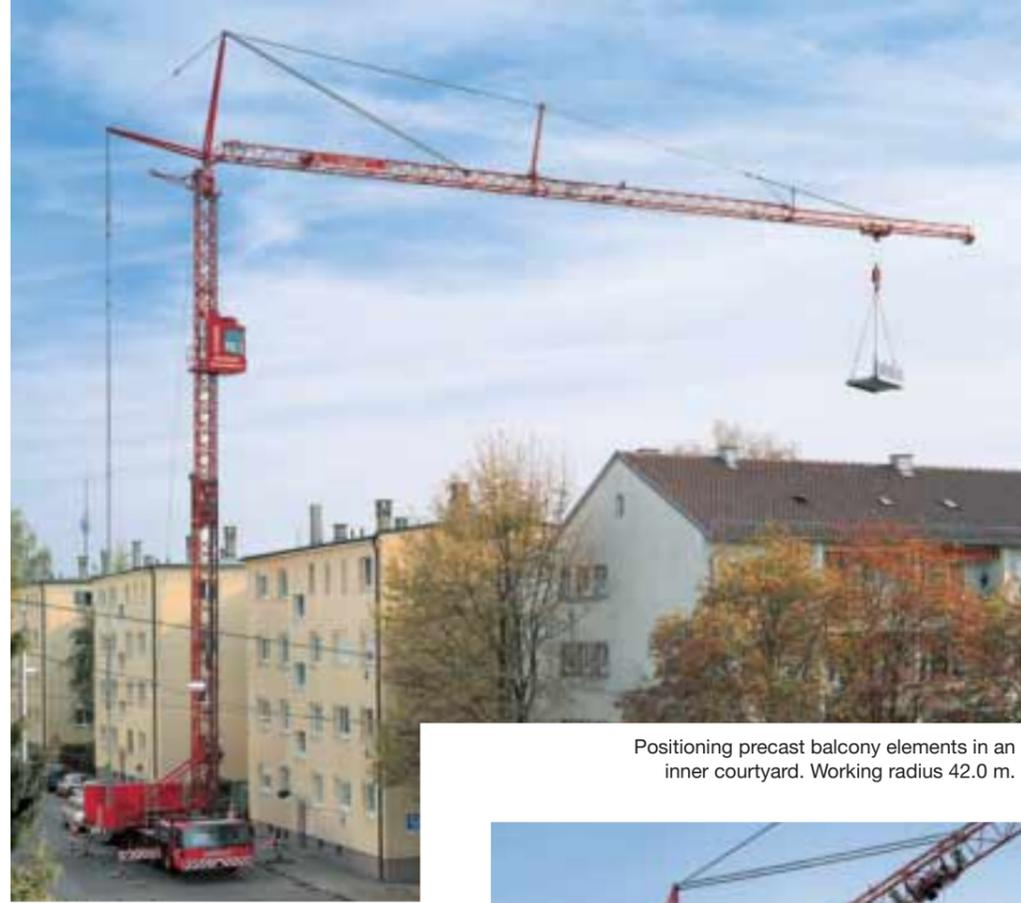
Positioning precast balcony elements in an inner courtyard. Working radius 42.0 m.
