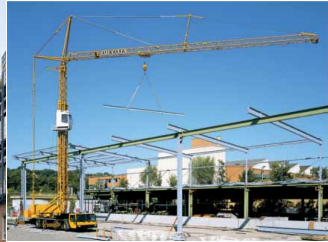
Crane operation with tower retracted.
